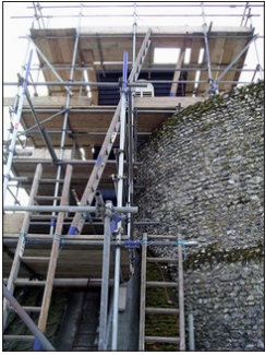
Work on the church funded by the Friends
